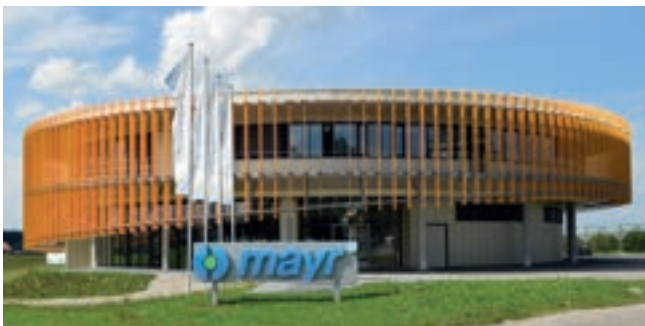
Communications Centre mayr.com – opened in 2018.
